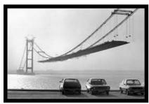
The Humber Bridge has a total length of just over 2200 metres, and a width of about 28 metres. The bridge was opened in 1981 and it cost nearly £100 million to build. The bridge was designed by Freeman Fox and Partners. The bridge is cleverly designed to bend more than 3 metres in heavy and winds.
