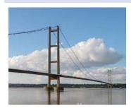
The Humber Bridge is a single-span suspension bridge. It spans the <u>Humber</u> (the estuary formed by the River Ouse and the <u>River Trent</u>). The bridge is made up three spans; Hessle side span (280 metres), Barton side span (530 metres) and the main centre span (1410 metres) making a total of 2200 metres or 1.4 miles. One side of the bridge is in Barton-upon-Humber, the other is in Hessle. The Humber Bridge has a larger span than the Golden Gate Bridge in the United States.
