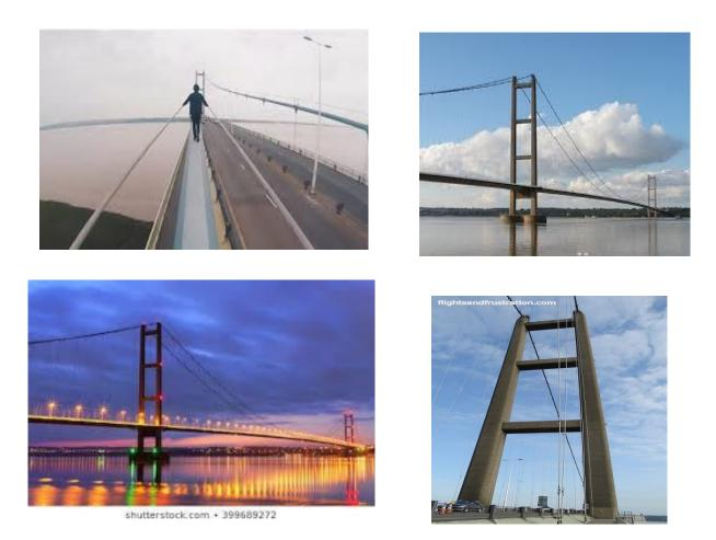
The Humber Bridge is a single-span suspension bridge. It spans the <u>Humber</u> (the estuary formed by the River Ouse and the <u>River Trent</u>). The bridge is made up of three spans; Hessle side span (280 metres), Barton side span (530 metres) and the main centre span (1410 metres) making a total of 2200 metres or 1.4 miles.One side of the bridge is in Barton-upon-Humber, the other is in Hessle. The Humber Bridge has a larger span than the Golden Gate Bridge in the United States.
